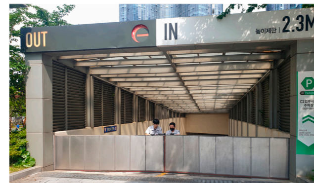
Facility Safety Inspection Site
